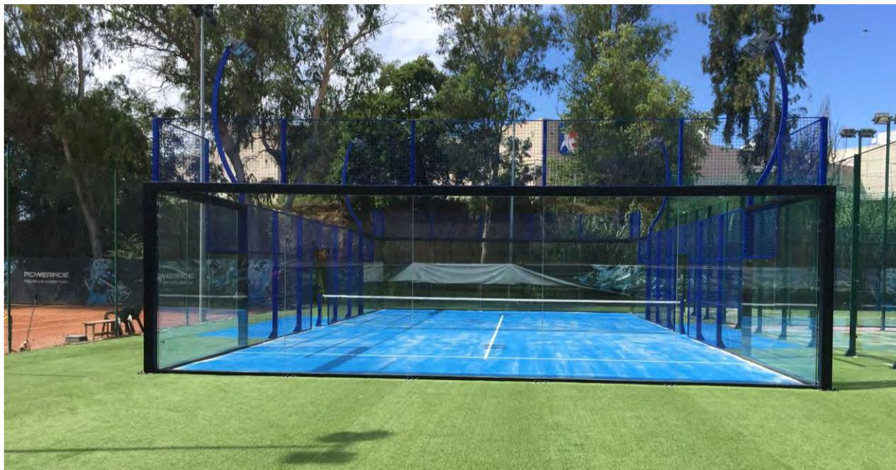
The side elevations will incorporate a central opening for player access on one or both sides, or where the out of court play area (8.00m x 2.00m overall) is to be incorporated for higher levels of play.
